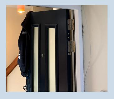
All doorset fitting and fixtures were pre installed from the manufacturer – ensuring the integrity of the fire door to it's 30 minute fire rating.
