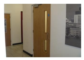
The other block also had a new FD30 door set installed to match the existing doors but also glazed partitioning by our engineers.
