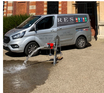
Fire hydrant inspection and annual wet testing
