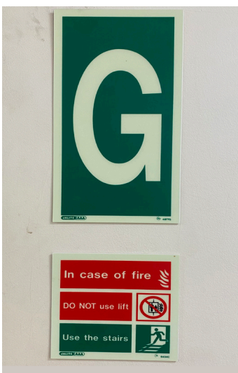
Installation of photoluminescent level signage in residential blocks of flats.
