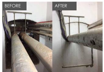
In the basement/server room to the bottom of the dumb waiter shaft there was a large opening with a number of pipes and cables passing through which needed to be sealed.
