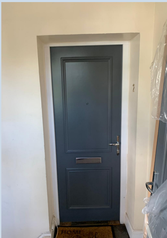
Replacement FD30s flat front door
