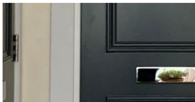
Following the fire stopping audit, new architrave was installed around doorsets
