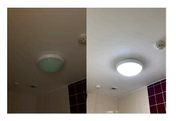
After the installation was completed, a function test was performed on each updated circuit and a certificate issued confirming that the Emergency Lighting was in working order.
