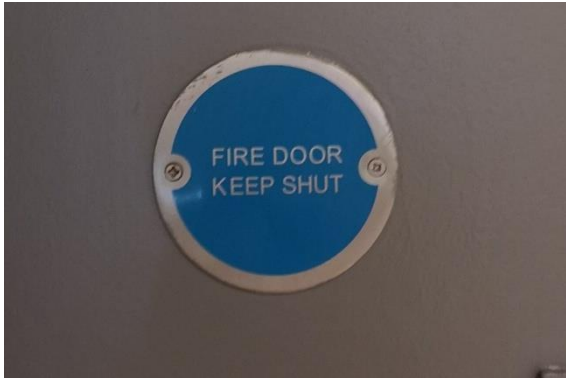
Fire door “keep shut” sign
